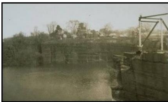
Portland quarry pit full of water 1928 – Connecticut Historical Society and Connecticut History Online. 30
