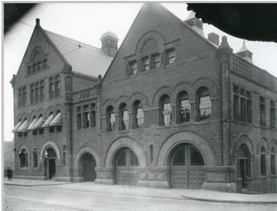
951-941 Boylston Street, The Police Station (left) and Fire Station (right) on the corner of Boylston Street and Hereford Street, October 17, 1911. 46
